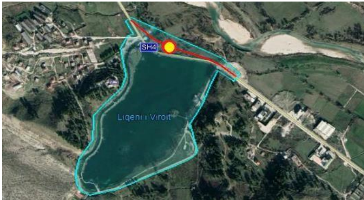
Figure 1. Existing and the new segment of the road.
